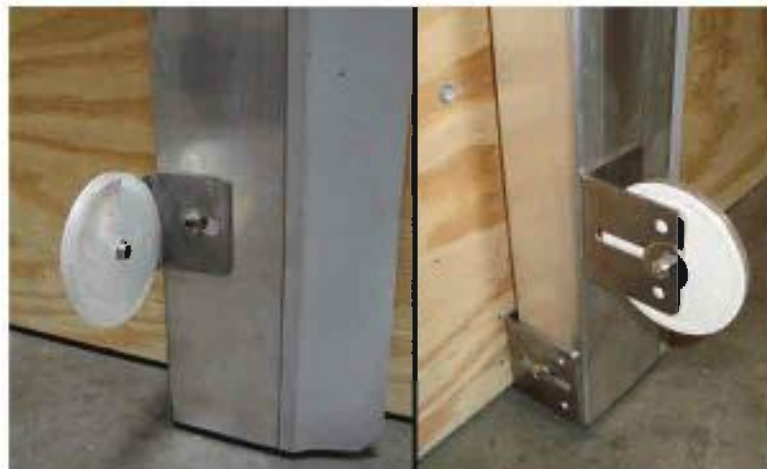
Photo #6 (Reflector Mounting)
