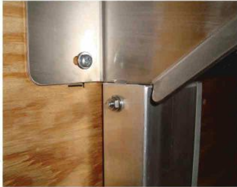
Photo #4 (Vertical Extrusion Orientation and Mounting)
