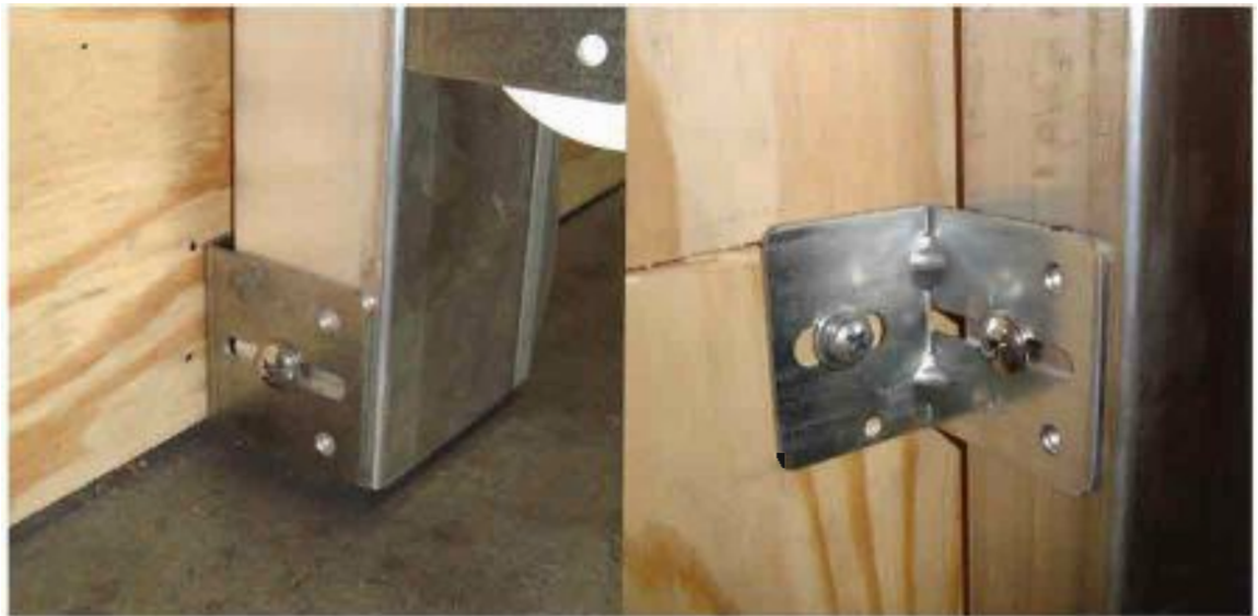
Photo #5 ("J" Bracket Mounting)
