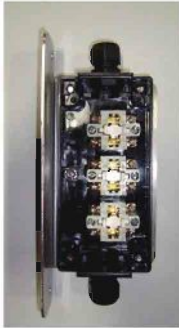
Photo #15 (NEMA-4 Preparation)
