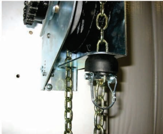
Photo #14 (Stop Bumper Installation)
