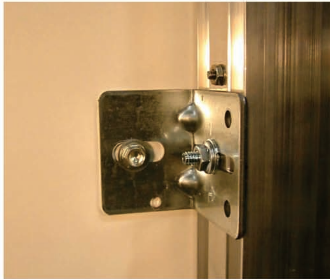
Photo #5 ("J" Bracket Mounting)
