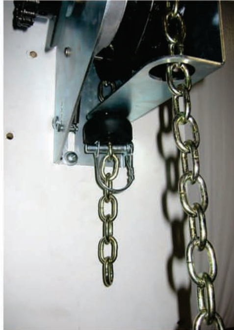
Photo #10 (Upper Stop Bumper Installation)
