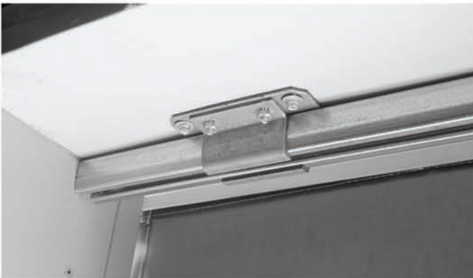
Photo #1 (Track and Splice Mounting)
