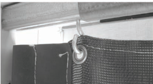
Photo #6 (Crimped Hanger Hook)
