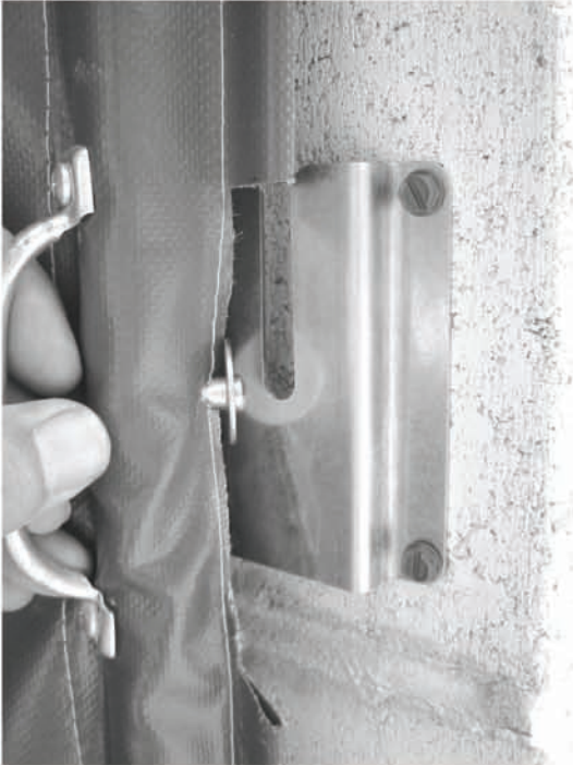
Photo #7 (Slot Lock Bracket Mounting)
