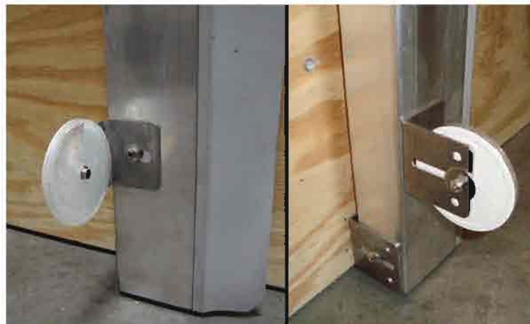
Photo #6 (Reflector Mounting)
