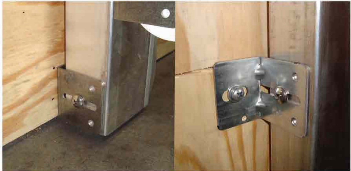
Photo #5 ("J" Bracket Mounting)
