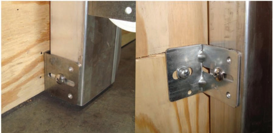
Photo #5 ("J" Bracket Mounting)
