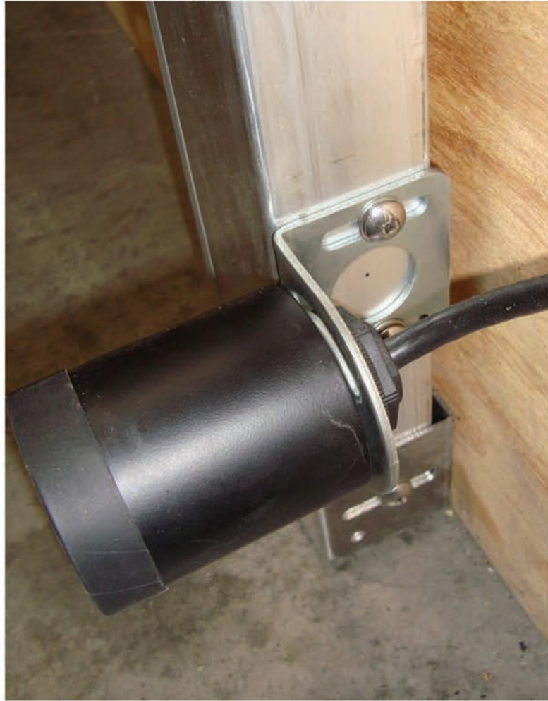
Photo #7 (Head Unit Mounting)
